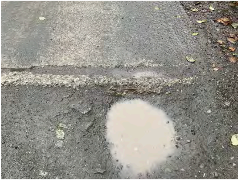
Right bank ballast wall
