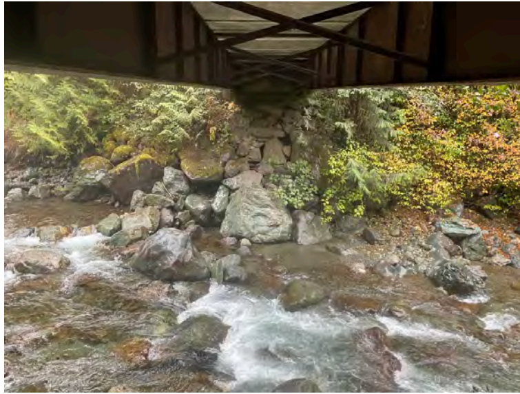
Left Bank Abutment when facing downstream
