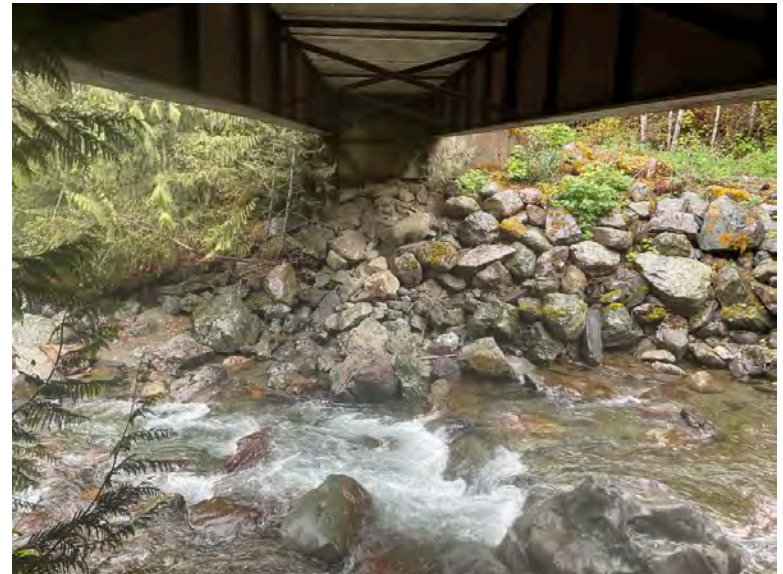
Right Bank Abutment when facing downstream
